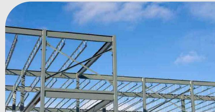
**Load zone joists** are installed in certain areas of the building in which more strength is required to provide support to the structure.
