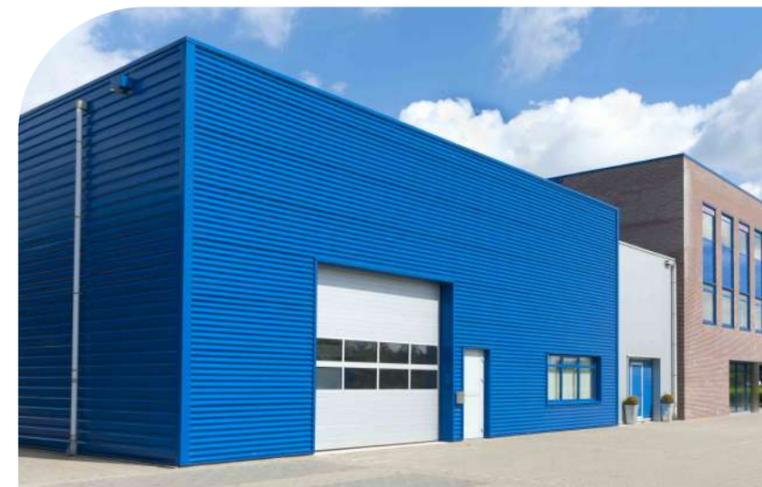
Hybrid projects combine the strong framework of metal structures with the efficient elements found in pre-engineered metal buildings. (PEMB) This creates a powerful and quick construction solution that marries durability with convenience. By integrating pre-engineered parts like panels and modular sections, these projects save time and money while delivering modern and adaptable structures.
