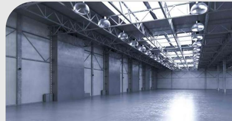
**Steel joist girders** are installed in roofs and floors to assist with the weight distribution of the structure. They are bolted to the columns and are installed fast and easily, which will also save you time and money on labor costs.
