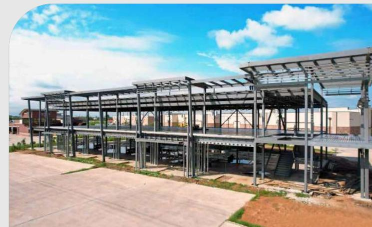
**Composite steel joists** are designed to help support the structure of the floors and roofs. They also provide additional strength and lessen vibration by adding a concrete slab. An advantage of this product is that it requires fewer columns and provides more space, saving you time and money you would need to spend on labor and supplies.
